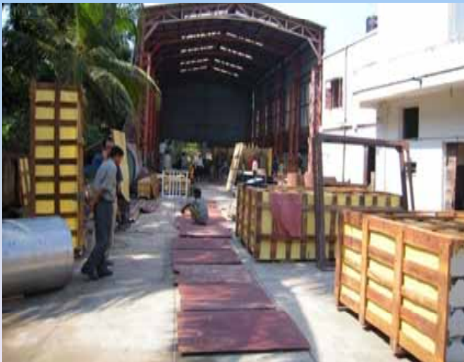
Fabrication of Accessories to Water & Effluent Treatment Systems
